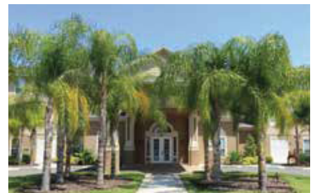
Lakeside Terrace Senior Apartments Winter Haven, FL Rental: 84 units AHP: $612,815 Total Development: $13,610,007
